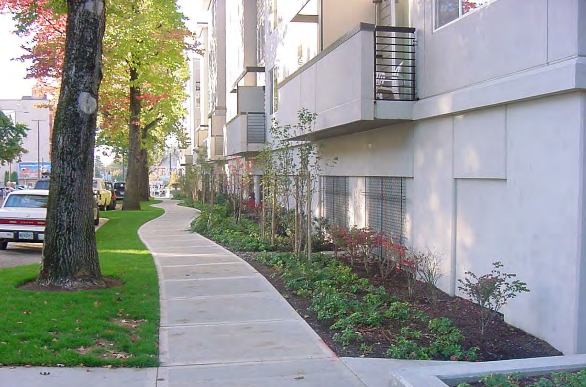
Buckman Terrace tree preservation and at grade infiltration planter (303 NE 16th Ave.)
