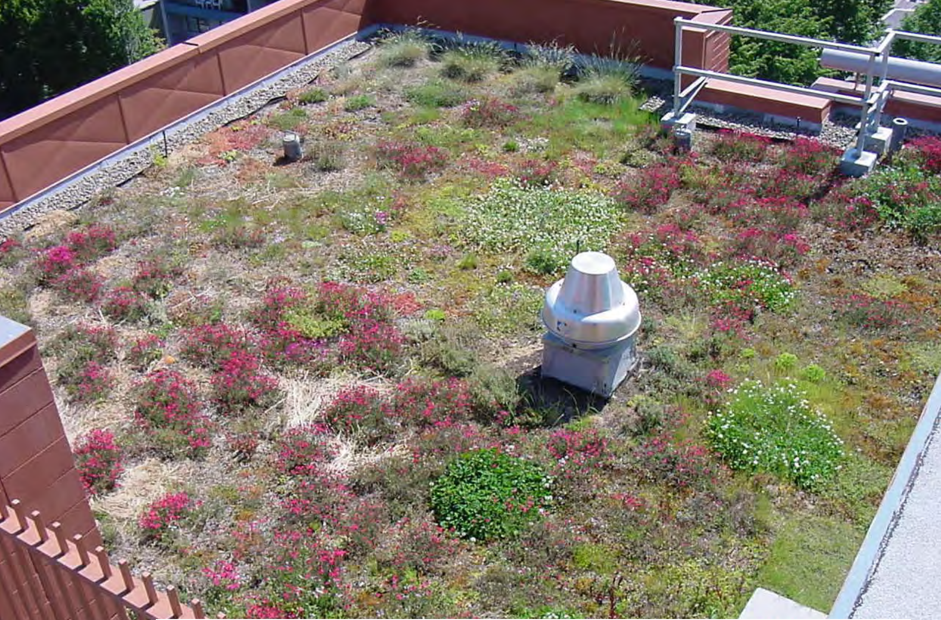
Hamilton Apartments Eco-Roof (1212 SW Clay St.)
