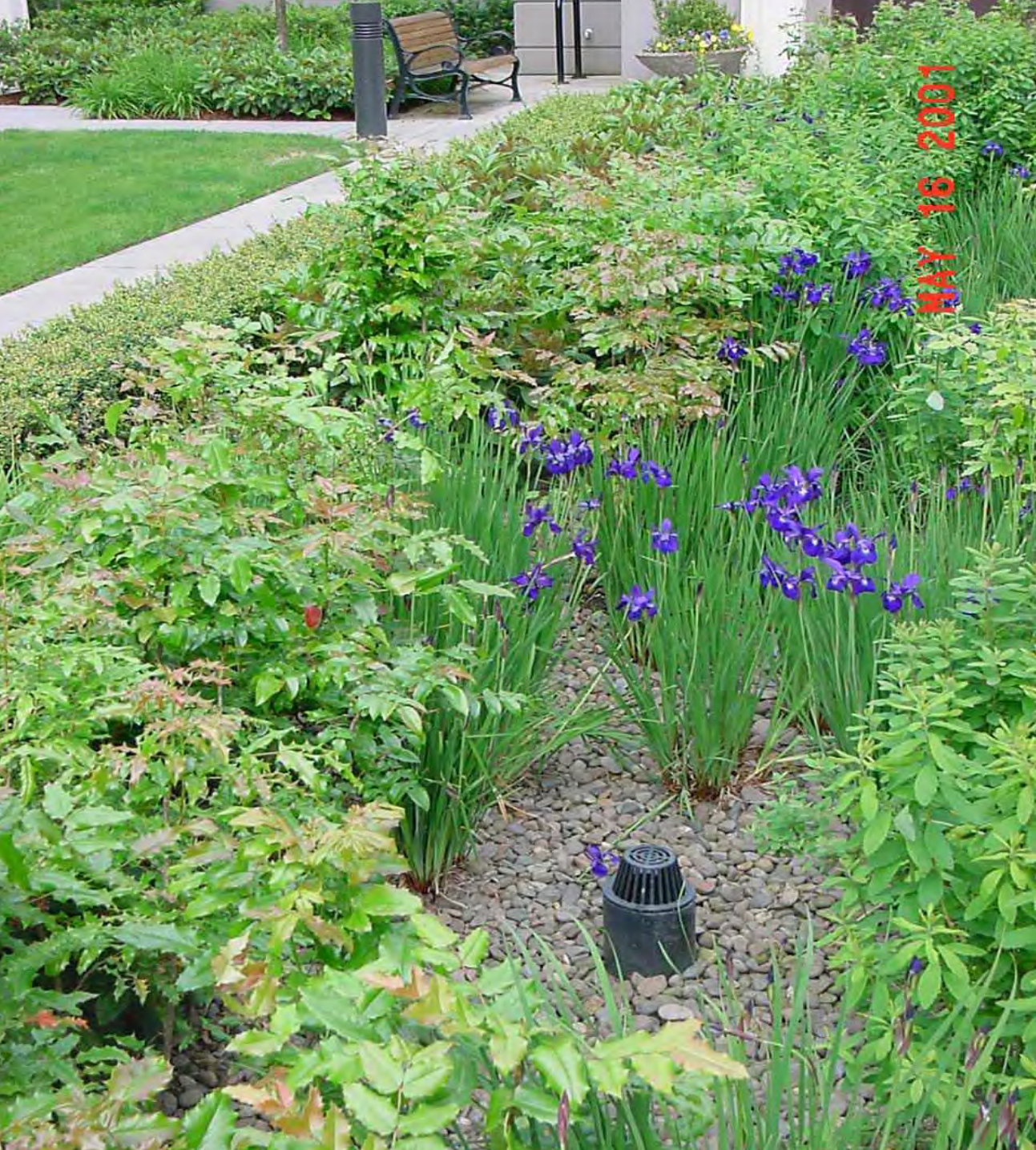
Buckman Heights courtyard planter overflow (430 NE 16th Ave.)
